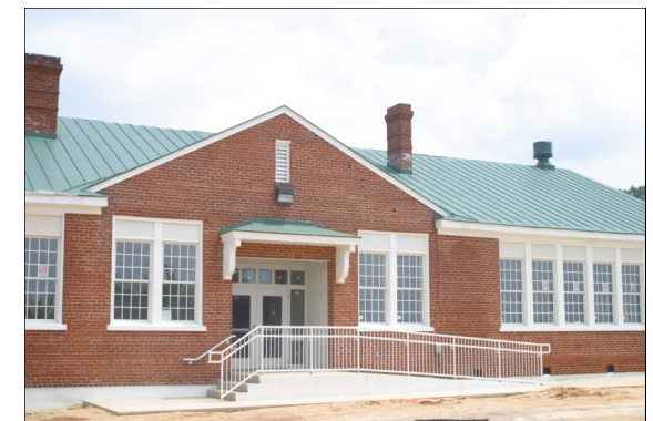
The newly renovated Russell Grove Building opened to alumni during the 2003 Reunion.
